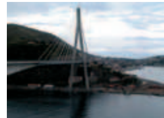
Figure 6.7 - The bridge over the Rijeka Dubrovačka.
